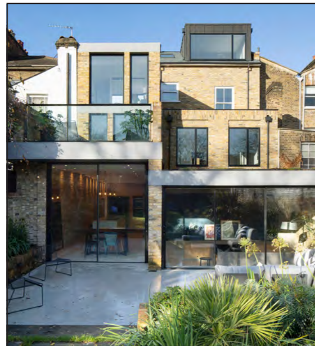
Fig. 70: Coach House in New Cross, designed by Selencky Parsons, is developed by one of the original land owner and delivers three flats and a new house (website: www.selenckyparsons.com , photography: Richard Chivers)
