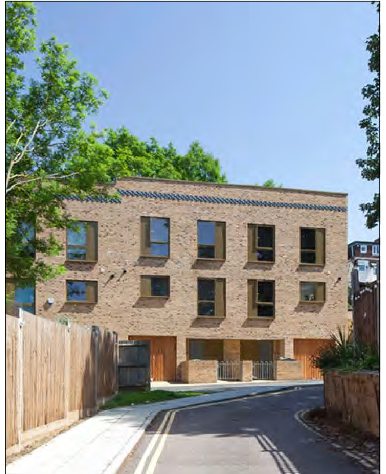
Fig. 91: New homes in Forest Hill designed by David Miller Architects (website: www.david-miller.co.uk , photography: TBC)
