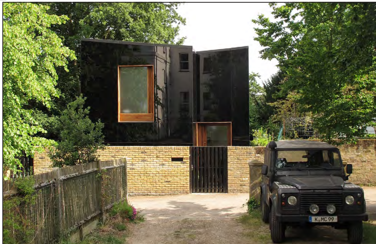
Fig. 76: This new home in Sydenham is designed using Passivhaus principles. It is designed by Ian McChesney Architects. (website: www.mcchesney.co.uk, photography: TBC)
