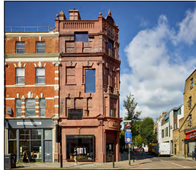
Fig. 136: This small site development in Islington is designed by Groupwork + Amin Taha. It references its surroundings in a contemporary way and includes a shop, show room and three apartments above. (website: groupwork.uk.com, photography: TBC)
