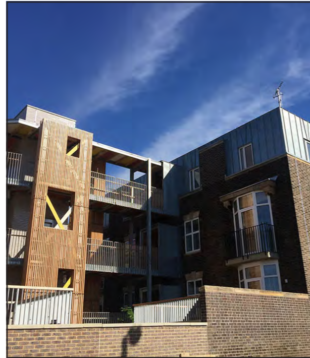
Fig. 158: The refurbishment and vertical extension of St Paul's House in Deptford by Ash Sakula (website: www.ashsak.com , photography: Ash Sakula)
