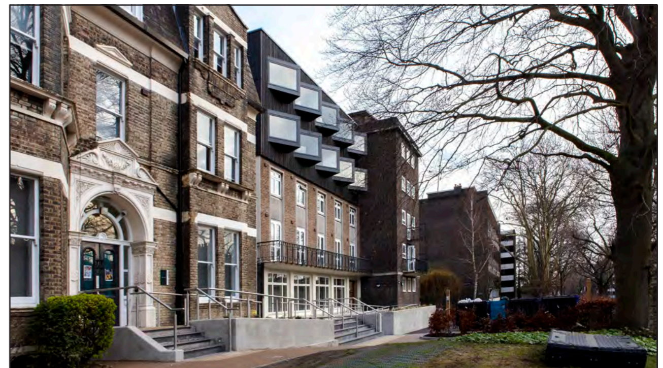
Fig. 157: Extension to Raymont Hall by Hawkins\Brown providing new student accommodation. (website: www.hawkinsbrown.com , photography: Francesco Montaguti)
