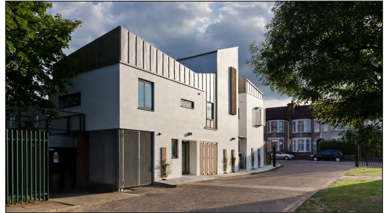
Fig. 134: The small residential development on the corner of two streets in Crofton Park replaces a school keeper's cottage with three flats and a small house. (website: www.chancedesilva.com , photography: Tim Crocker)
