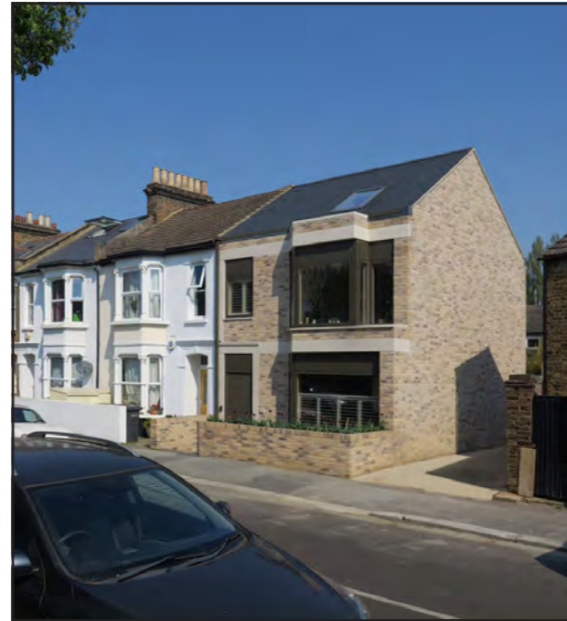
Fig. 118: Replacing disused garages, House on the End by architect 1200 Works extends an existing Victorian terrace to create a new family home. (website: www.1200works.com, photography: TBC)
