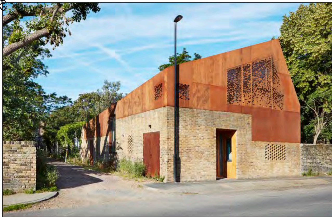
Fig. 124: This new house by Stolon Studio cleverly utilises a site at the entrance to an existing mews to create an attractive family home. The front door is set back from the pavement and ground floor windows use hit-and-miss brickwork to provide privacy. (website: www.stolon.co.uk , photography: TBC)
