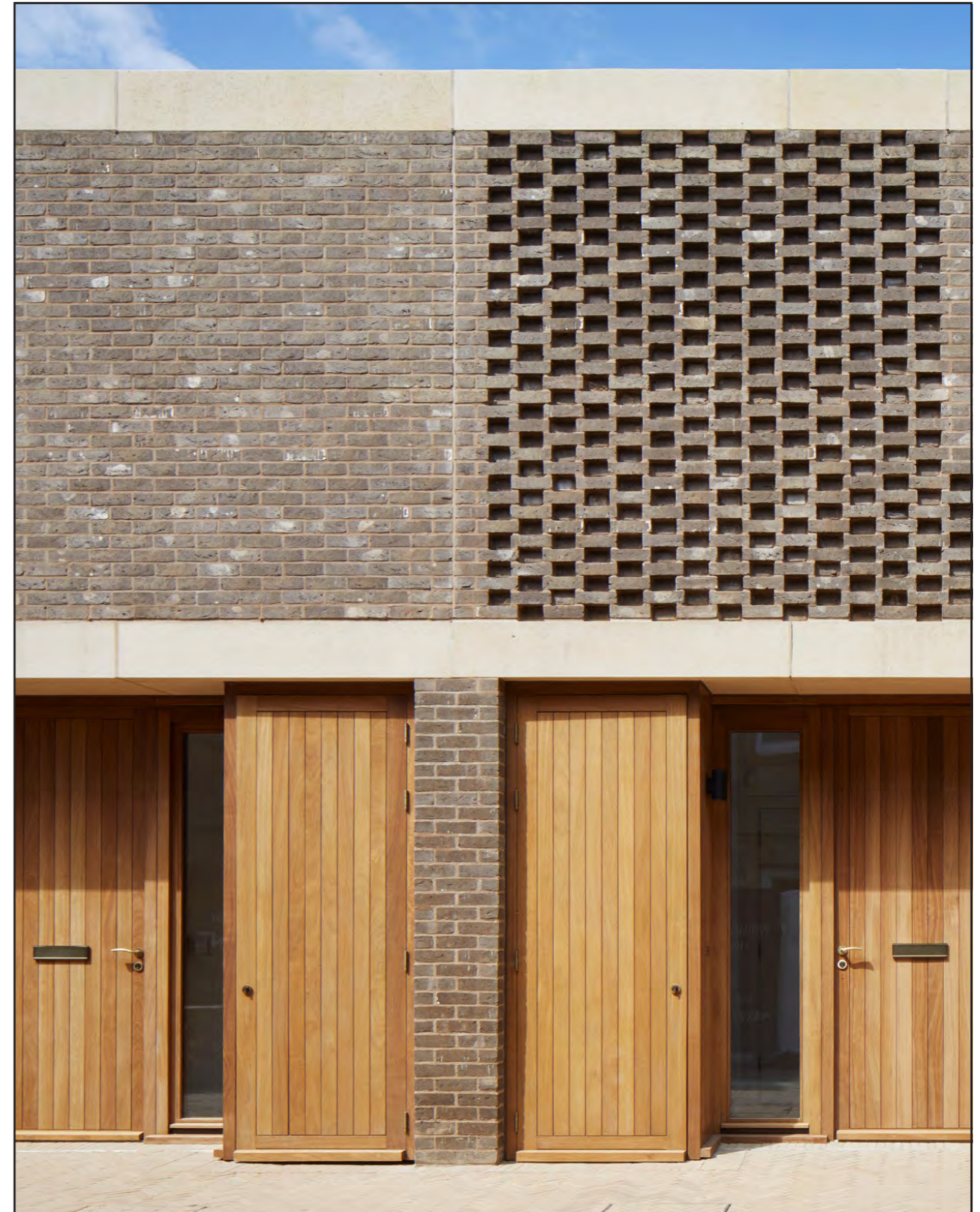
Fig. 32: These new mews houses in Sevenoaks, designed by Morris + Company, smartly integrate waste storage into the building envelope, providing a more friendly and usable public realm (website: www.morrisandcompany.com , photography: Jack Hobhouse)
