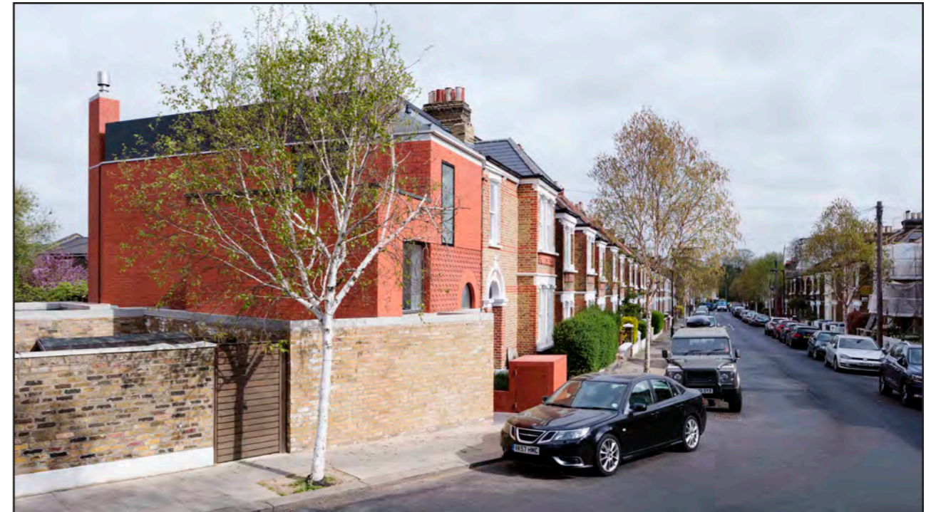
Fig. 122: Respecting the height and detail of the neighbouring houses, this new family home by 31/44 architects extends an existing Victorian terrace in Southwark. (website: www.3144architects.com , photography: Rory Gardiner)
