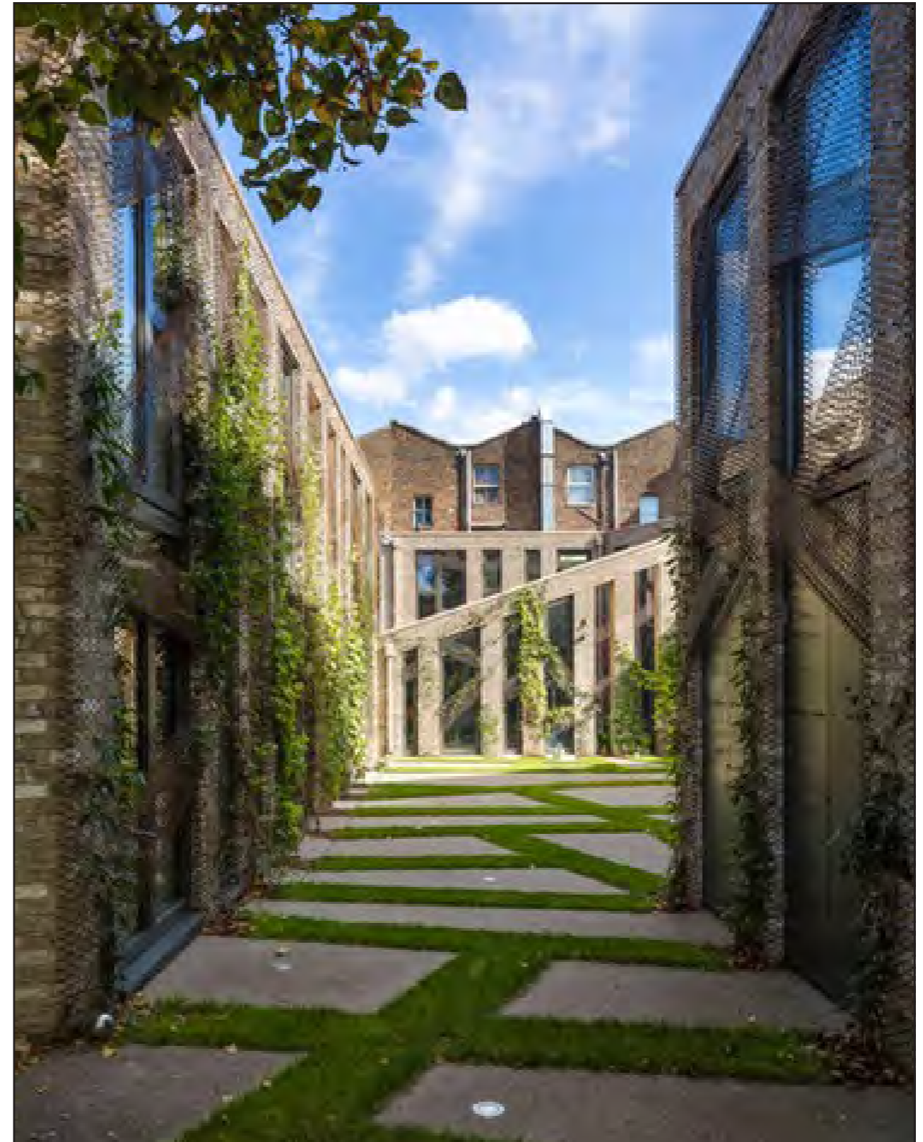
Fig. 34: Access into Forest Mews, designed by Stolon Studio, is via a private road which allows soft landscaping to be integrated into the vehicular access (website: www.stolon.co.uk , photography: Robert Baker)
