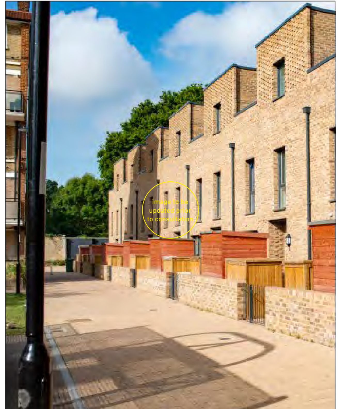
Fig. 16: New Homes at Longfield Crescent in Forest Hill designed by Pollard Thomas Edwards Architects (website: www.pollardthomasedwards.co.uk , photography: TBC)
