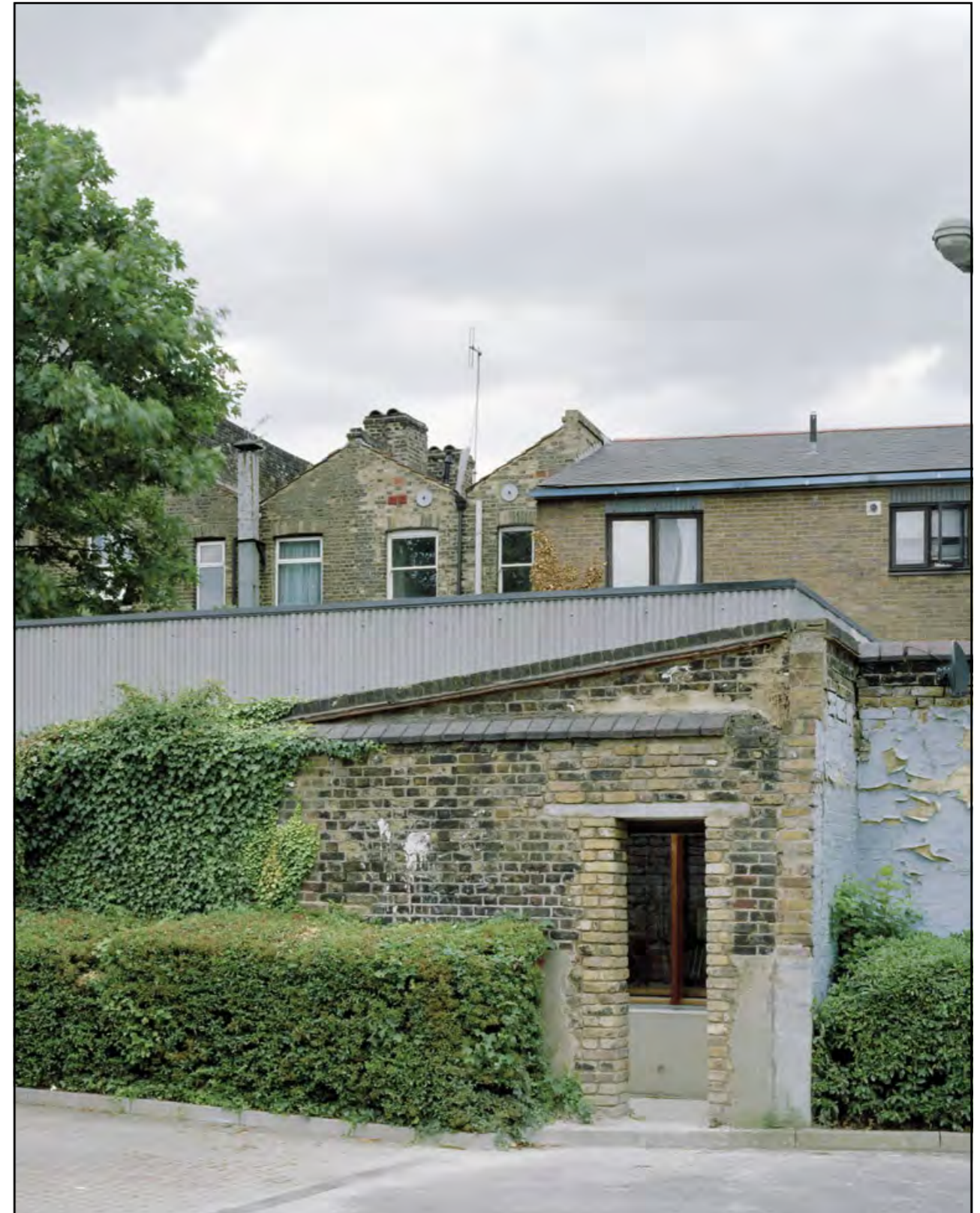
Fig. 87: Strange House designed by Hugh Strange Architects in New Cross (website: www.hughstrange.com , photography: TBC)
