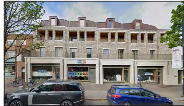
Fig. 163: Vertical intensification in Southwark designed by Panter Hudspith (website: www.panterhudspith.com, photography: Panter Hudspith)
