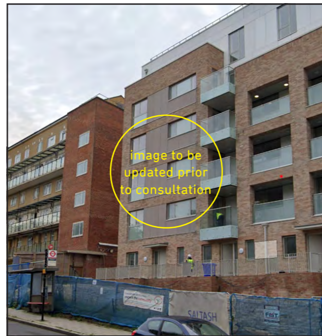
Fig. 102: Forster House in Whitefoot designed by Levitt Bernstein Architects (Website: www.levittbernstein.co.uk, Photography: NEEDED )
