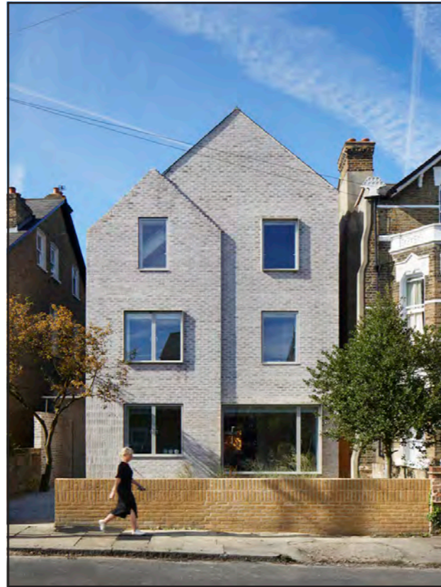
Fig. 184: Vertical extension and re-cladding of an existing house following the principles of Street Infill development. Designed by Alma-nac (website: www.alma-nac.com, photography: TBC)
