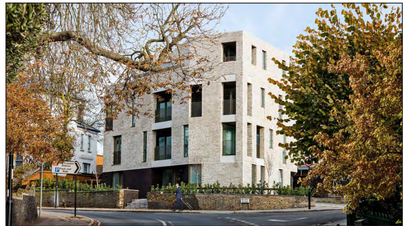
Fig. 135: This development in Croydon by OB Architecture creates a striking, high-density residential development on a prominent corner, with a building taller than its neighbours. (website: obarchitecture.co.uk , photography: Martin Gardner)
